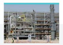
Provisioning injection water to the oil fields of southern Iraq, run by South Oil Company. The oil fields will use the seawater for enhanced oil recovery, where water is injected into the reservoir, allowing for increased oil production. **Client: Ch2m Hill**
